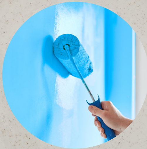
PAINTING / ELECTRICAL WORK
